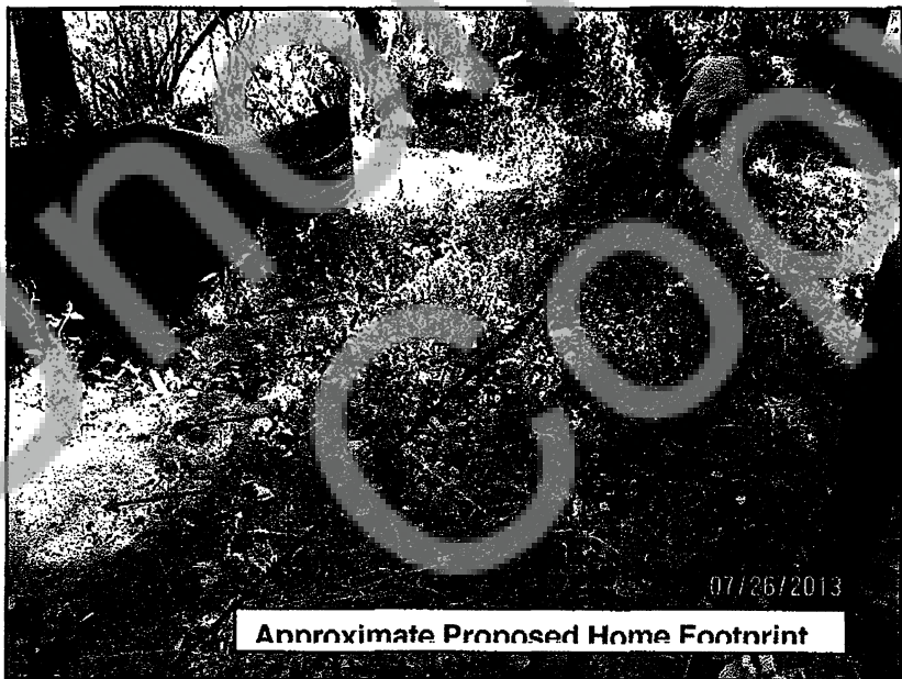
Photo 2: Approximate northeast corner of proposed home as observed on July 26, 2013. The hashed red line indicates the fill mass that has slowly settled and crept laterally down the slope.
