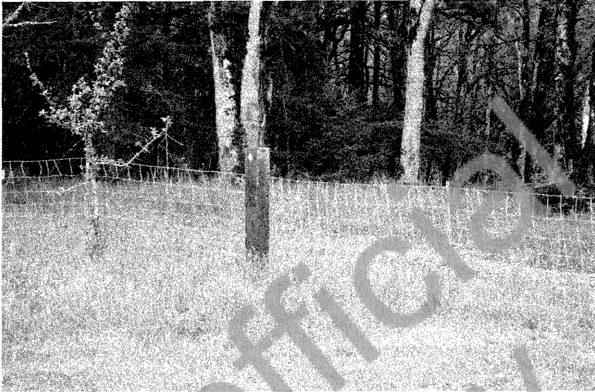
Photograph 1. Example of acceptable fencing within core habitat areas using wood and metal posts and woven wire fencing with a 6-inch by 7-inch mesh size.
