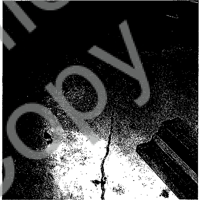
Photograph 4: Interior garage slab crack near south wall.
